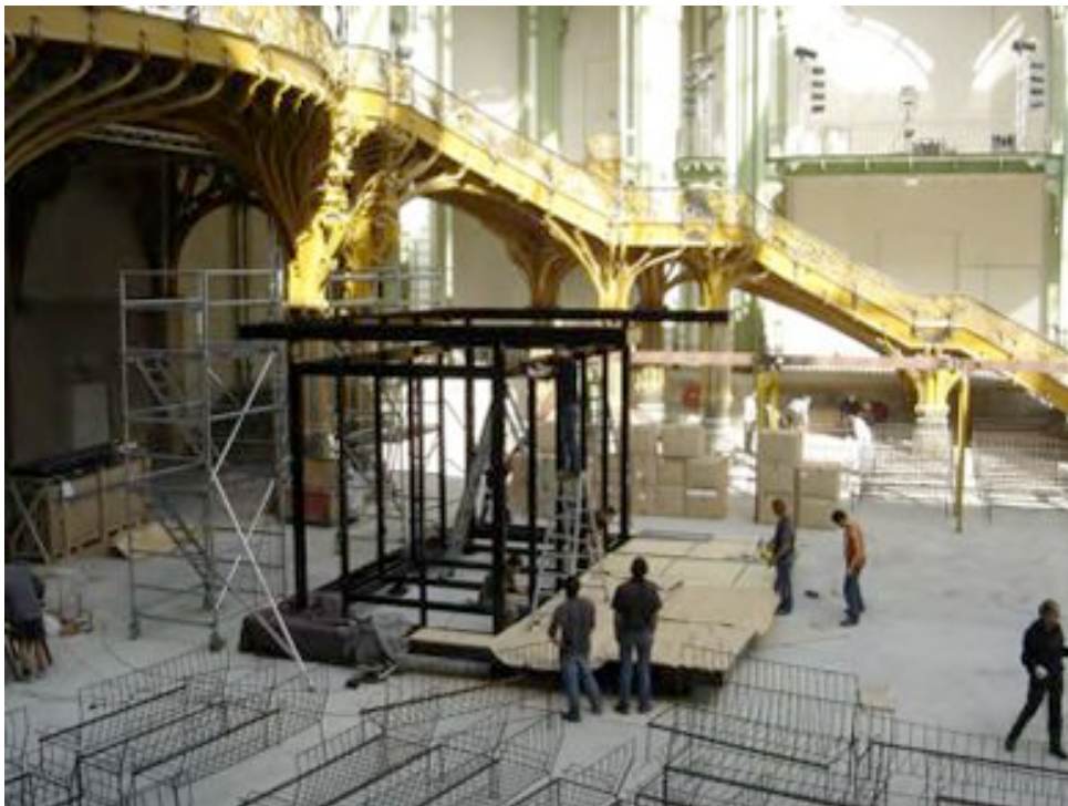
MONTAGE IN SITU
