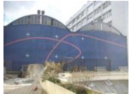
FACADE ETAT INITIAL
